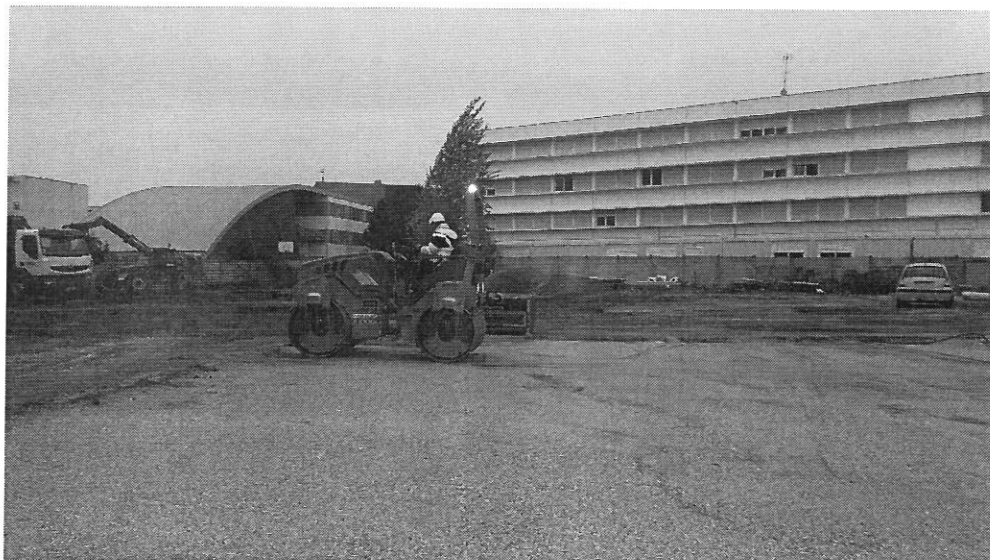
Figure 19: Compactage des fouilles
